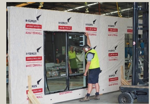
External walls with windows installed
