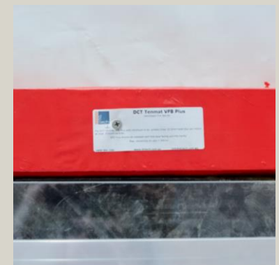
Cavity barriers as required
