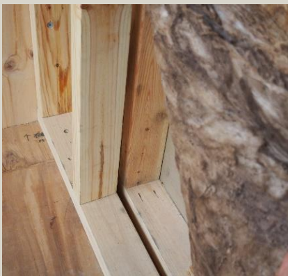
Discontinuous stud wall frame
