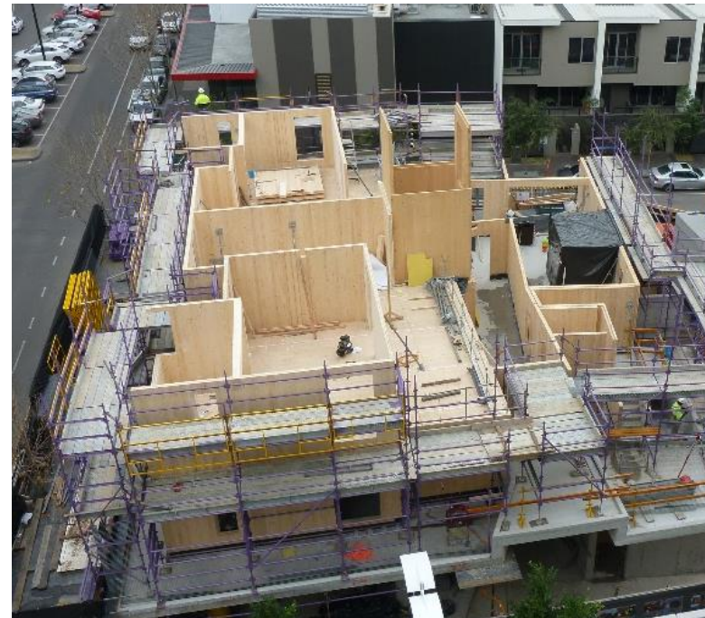
Massive CLT panels being installed over a first floor concrete podium
