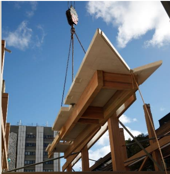
Prefabricated timber-concrete composite floor panel
