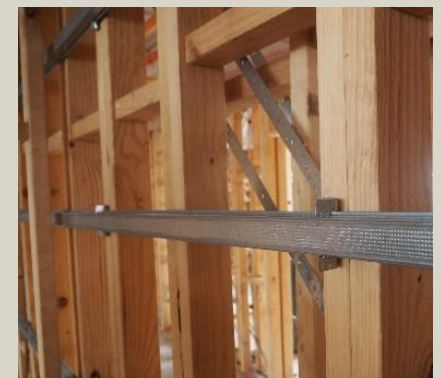
Single stud walls with resilient supports
