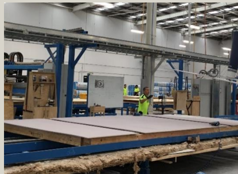
Wall lining installation
