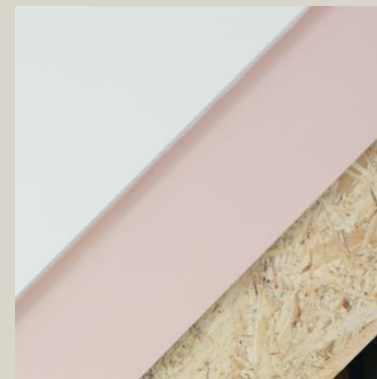
Encapsulated timber structure
