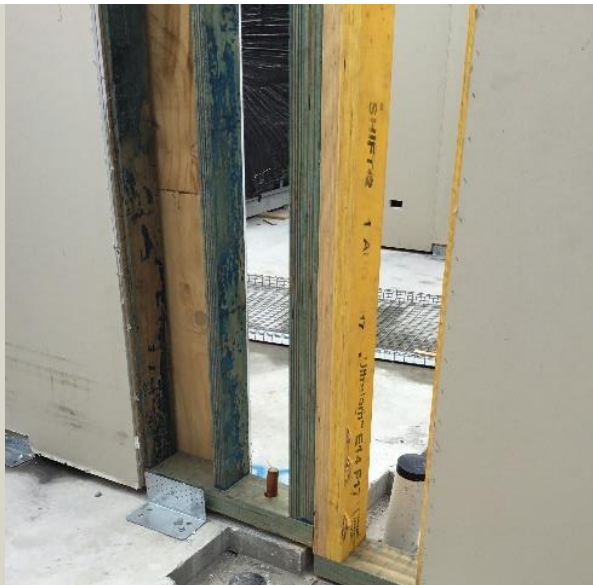
Offsite fabricated panelised lightweight timber framed wall systems
