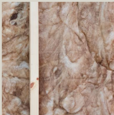
Non-combustible insulation
