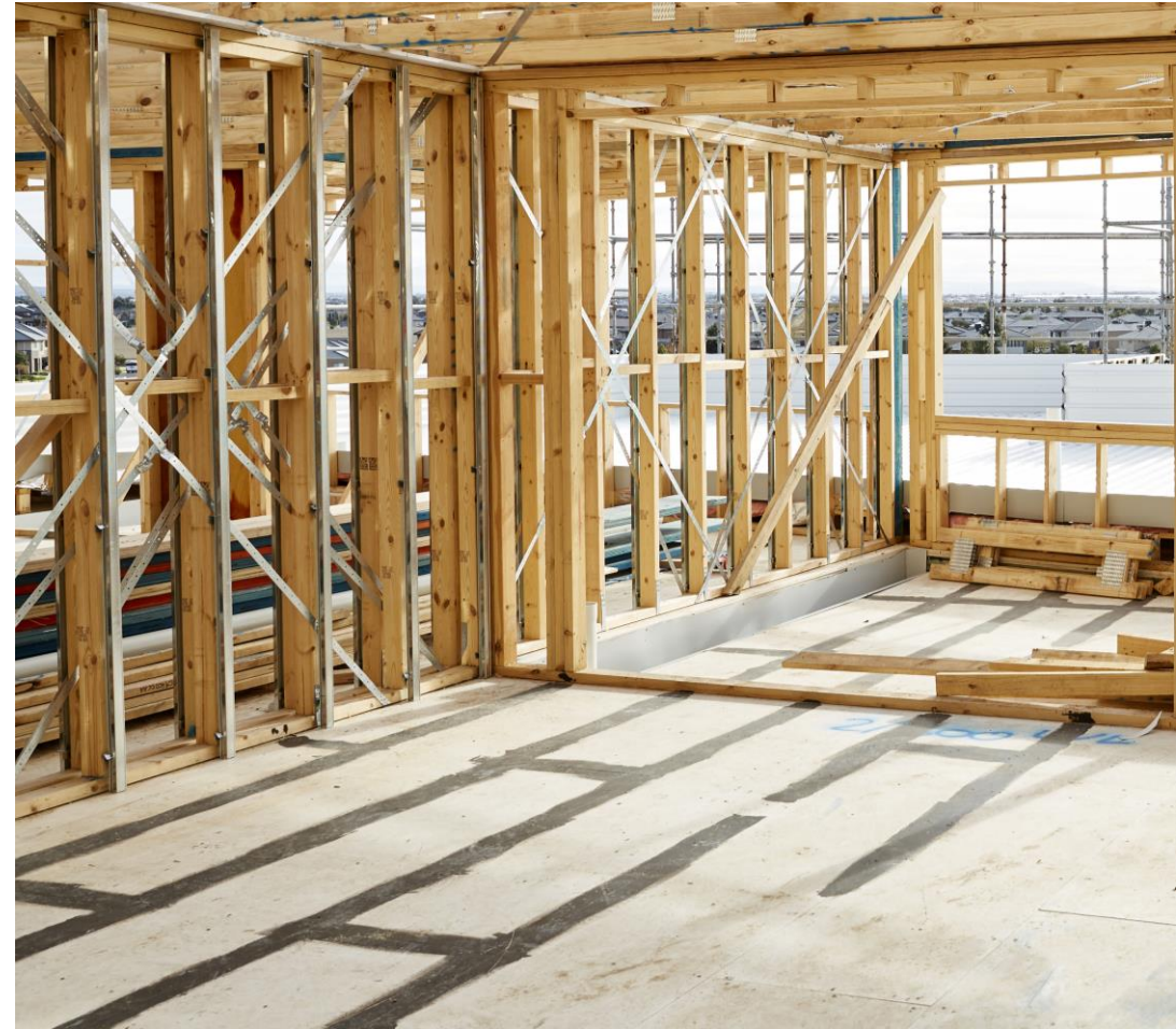
High performance wall and floor acoustic systems prior to concealment with finishing boards. Resilient-mounted furring channel can be seen installed directly to the loadbearing studs, while a form of cement sheet product has already been installed on the floor (black lines indicate where joints have been waterproofed).
