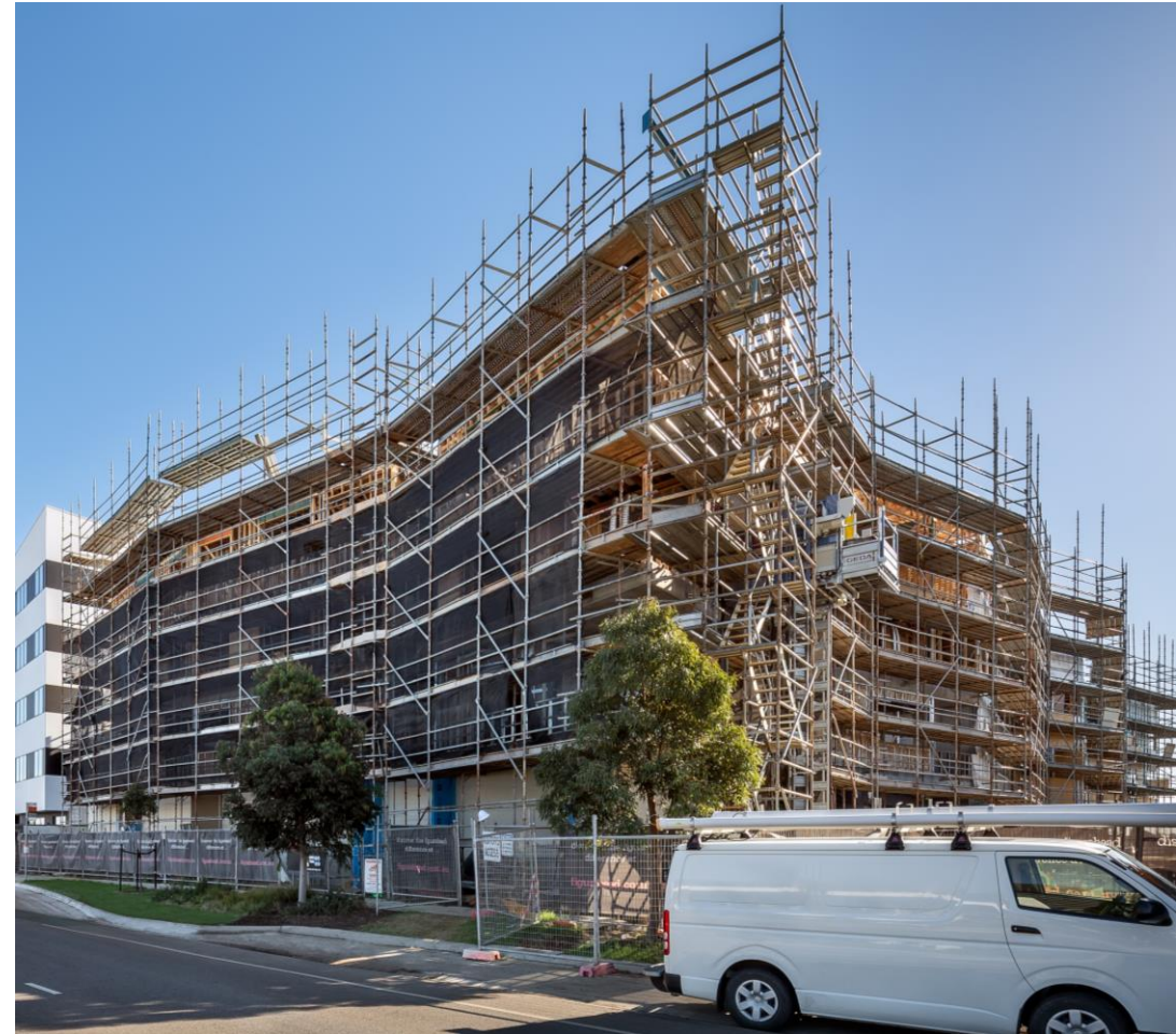
The Oxford Apartments utilized an insitu reinforced concrete structure for the ground and first floor, with timber structure for all floors above this. Here concrete was utilized to provide effective separation between the main Class 2 structure and the Class 7a car park.
