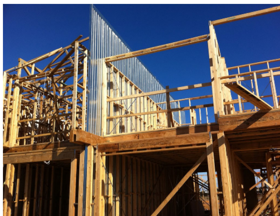
(a) Speedpanel separating wall
