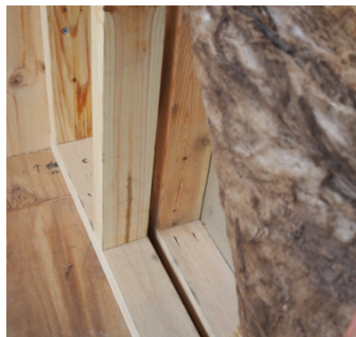
Figure 1: Double stud timber-framed separating wall.
