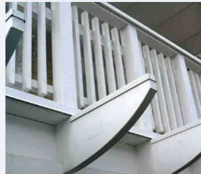
Capping protects top and end grain of projected beam.
