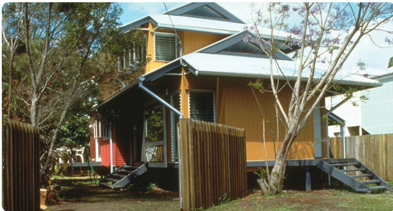
Large overhangs provide good protection.
