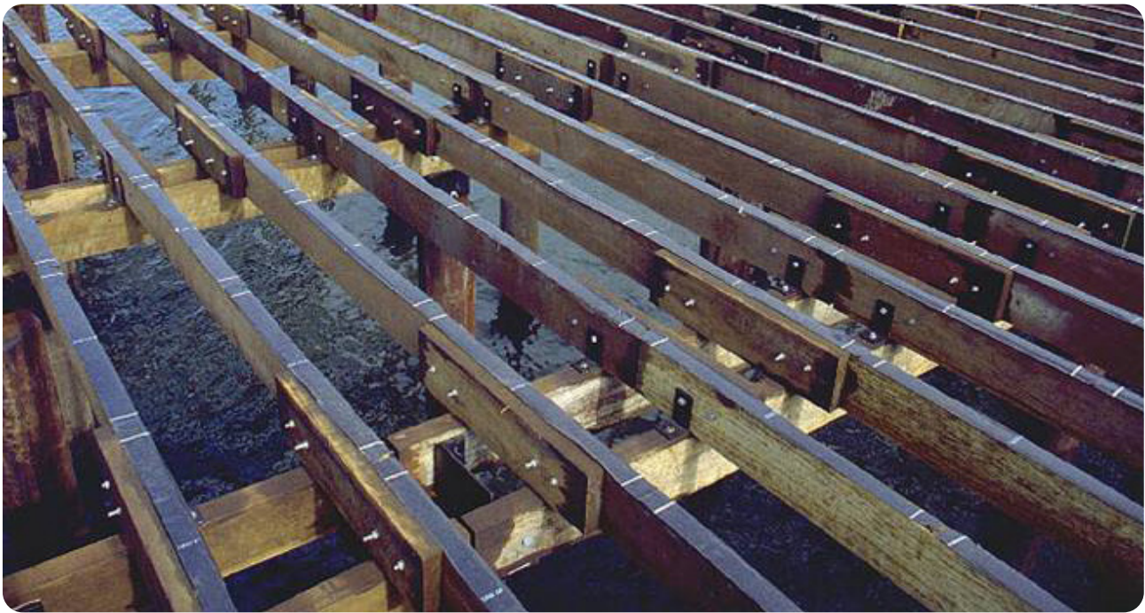
Bituminous DPC fixed to top of deck joists.
