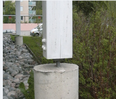
A well-ventilated, free-draining post support.
