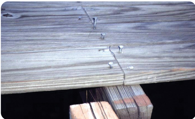
Plain shank decking nails in pine have ‘worked out’ with cyclic wetting and drying.
