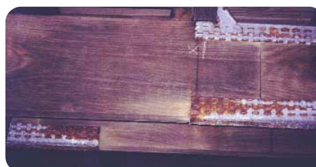
Corrosion of nail plates on deck joists after 6 years exposure near surf beach.
