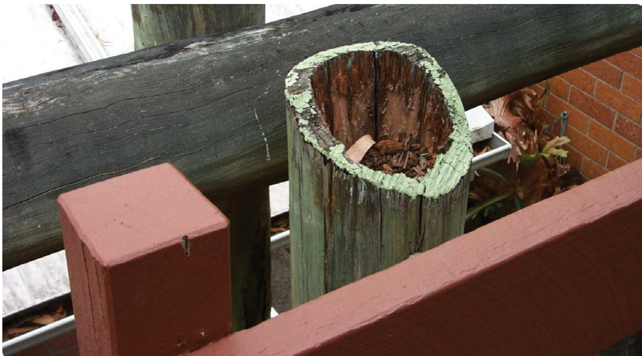
CCA treated sapwood outperforming durability class 2 heartwood.
