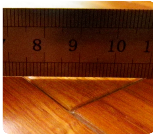
Figure 7.4: The effect of bevelled edges minimising mismatch effects.
