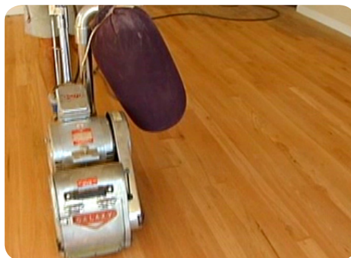
Figure 8.6: The finish sand.
