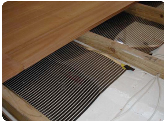
Figure E3: Blackbutt flooring (130 mm wide) with electric underfloor heating in Adelaide.
