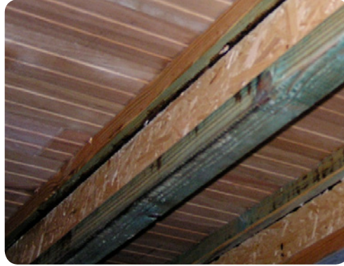
Figure 4.7: Timber floors are successfully laid over a range of solid timber and engineered joist systems.
