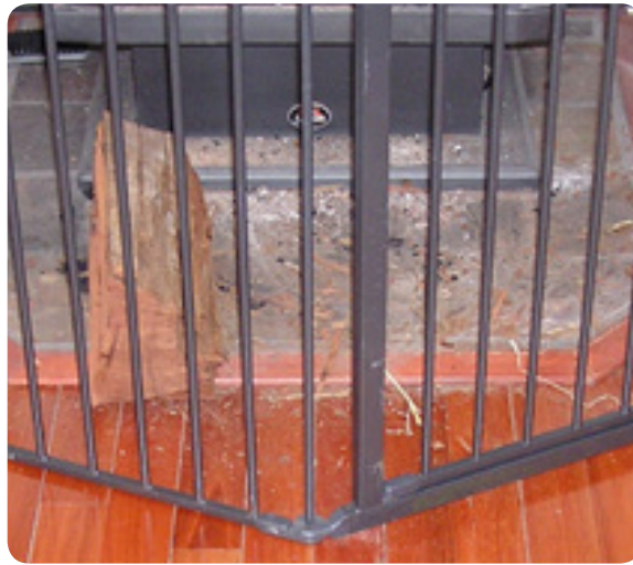
Figure 3.11: Intense heating sources can cause localised shrinkage.
