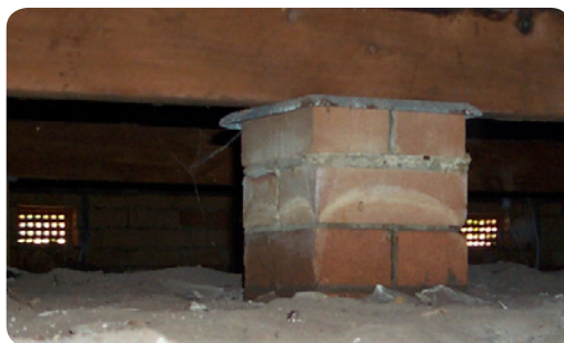
Figure 3.15: A dry sub-floor space and adequate ventilation is essential for floor performance.
