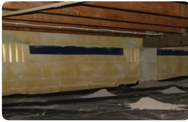
Figure 3.20: For frequently damp soil conditions, the sub-floor ground level can be raised with crusher dust and a polyethylene membrane laid over it.
