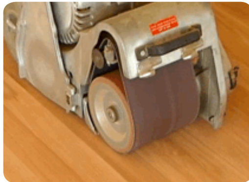
Figure 8.4: Third pass of sanding in the board direction.
