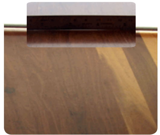
Figure 9.4: Cupping – Board edges higher than the centre of the board, but which is barely visible in the floor.
