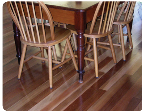
Figure 5.1: Spotted Gum direct stick overlay floor.
