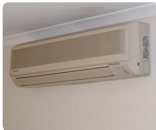
Figure 3.13: In warm climates these units are referred to as reverse cycle split system refrigerative air conditioners. In cold climates such as New Zealand they are referred to as heat pumps.
