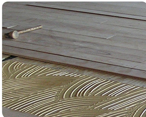
Figure 4.20: Adhesive spread prior to fixing.
