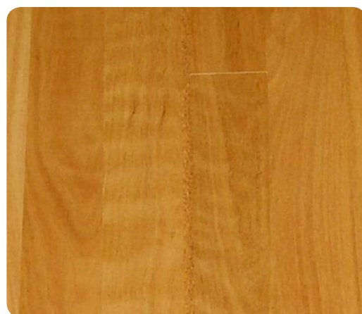
Figure 4.3: Cork intermediate expansion joints blend in well with timber floors.
