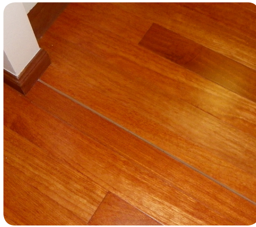
Figure 7.5: Caulked joint used to relieve potential expansion pressure through a narrower doorway linking two larger floor areas.
