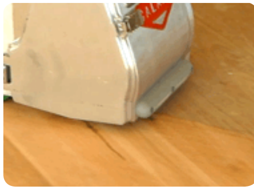
Figure 8.3: First and second pass of sanding at 45° to board direction.
