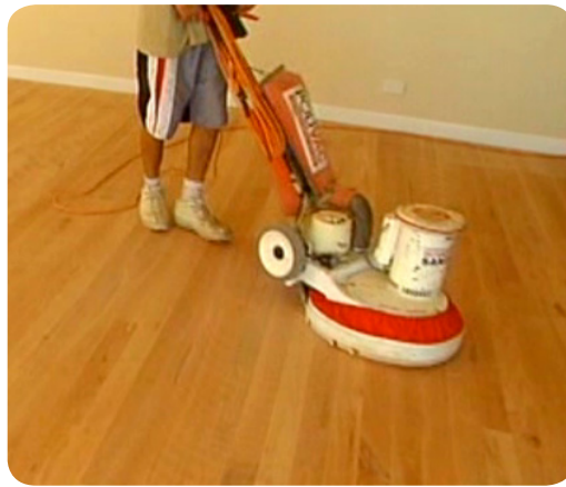
Figure 8.8: Buffing the floor.
