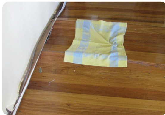
Tenting of T&G floor due to prolonged moisture being trapped under the floor. This inundated T&G floor supported on a particleboard sub-floor 'tented' about one week after the flood water receded.
