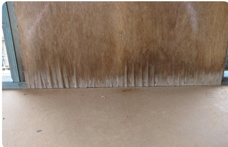
Plywood delamination at bottom plate in bracing panel. Note: The plywood used in the construction in the above example had no identification stamps or indication of certification schemes or Australian Standard for its manufacture.
