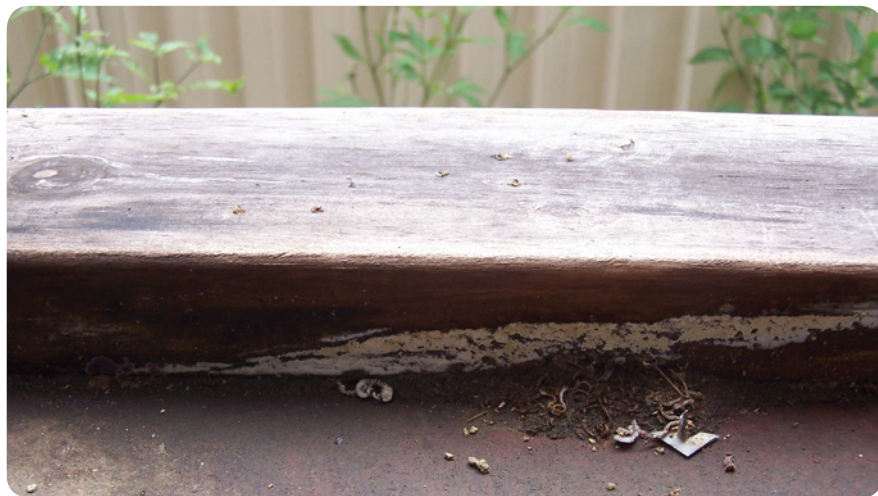
Decay in bottom plate on particleboard floor. Note small drill holes on top of plate used to detect decay.
