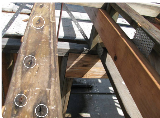
Decay pockets (highlighted) around fixing points where sheet flooring has been removed after 12 months' weather exposure.
