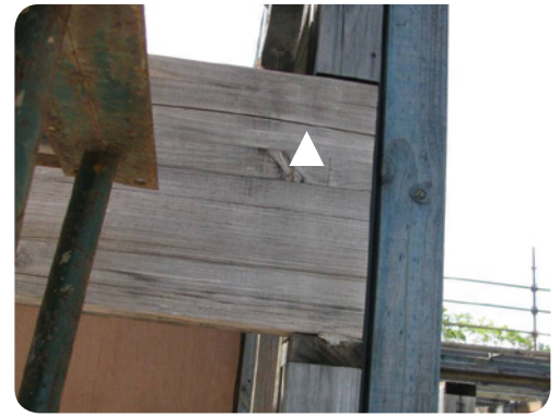
Split (indicated by arrow) along second top laminate (does not follow glue line) at end of beam.
