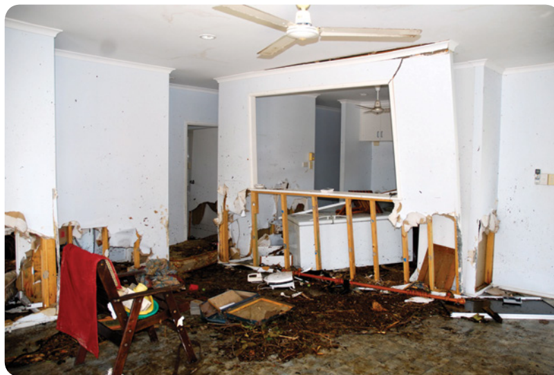
Storm surge structural damage. (Image: Cyclone Testing Station, James Cook University, Townsville)
