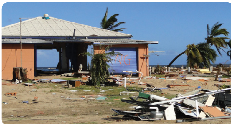
Storm surge damage to a slab on ground house. (Image: Cyclone Testing Station, James Cook University, Townsville)
