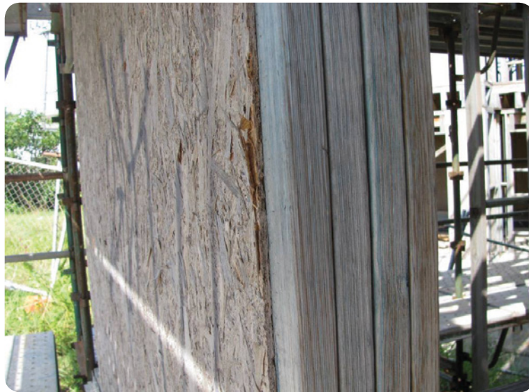
Example of OSB sheet bracing showing edge swelling and flaking.
