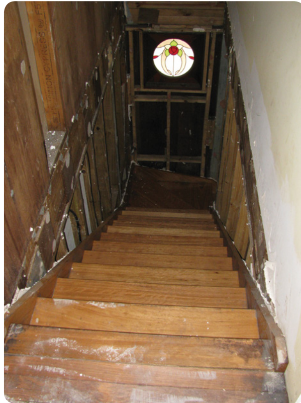
Solid timber stairs stripped out and allowed to dry were recovered following inundation.
