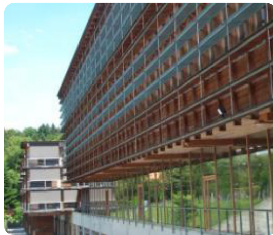
Figure 11: Sheltered bare timber.
