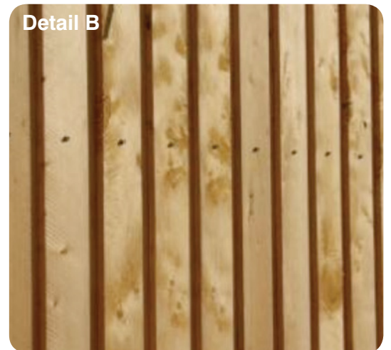
Figure 22: Visually significant fasteners; vertical green timber cladding.
