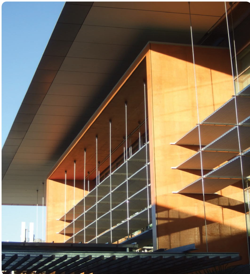
Figure 6: Stained and coated external plywood cladding.
