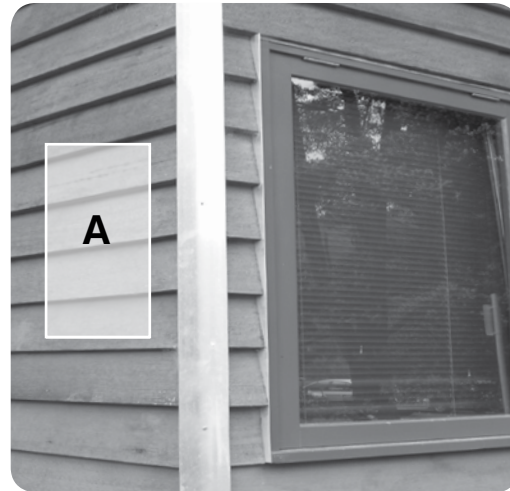
Figure 21: Detailing green timber weatherboards to allow movement.
