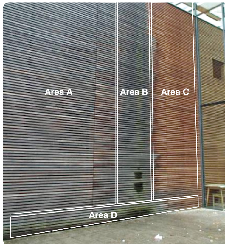
Figure 10: Differential weathering across a façade.
