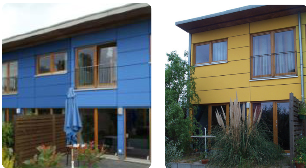
Figure 7: Painted plywood cladding, varnished timber joinery.
