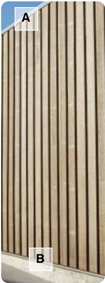
Figure 15: Detailing to avoid standing water.
