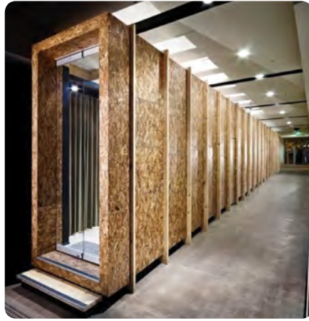
Matt Gibson Architecture and Design: The Coop - structure and cladding constructed from LVL Beams and OSB Panelling.
