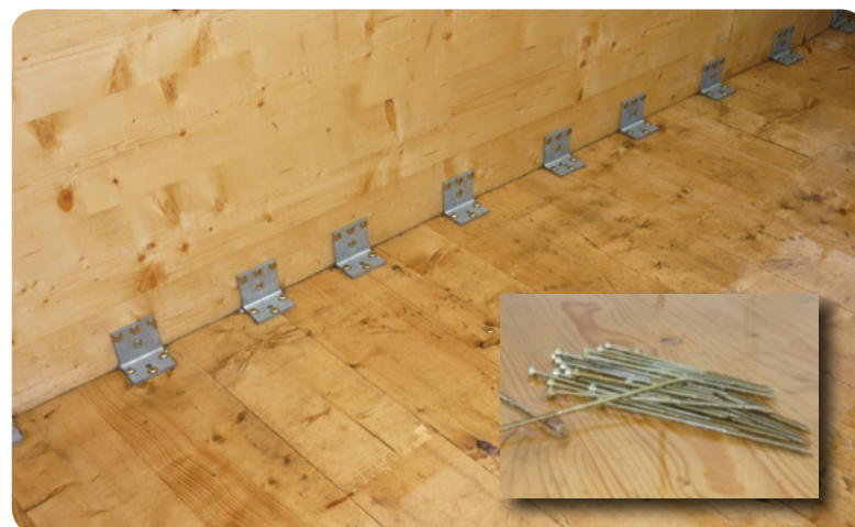
Figure 5.4: Wall to floor connection. Photograph: TDA
