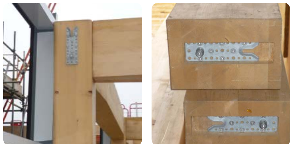
Figure 5.5: Specialist Timber Connector. Photograph: TDA
