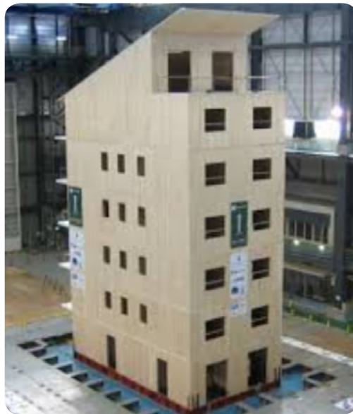
Figure 6.4: 7 storey CLT building on a shake table
