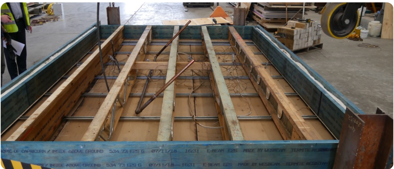
Figure 111: Upper surface of floor cavity with flooring removed showing no visible damage to the floor.
