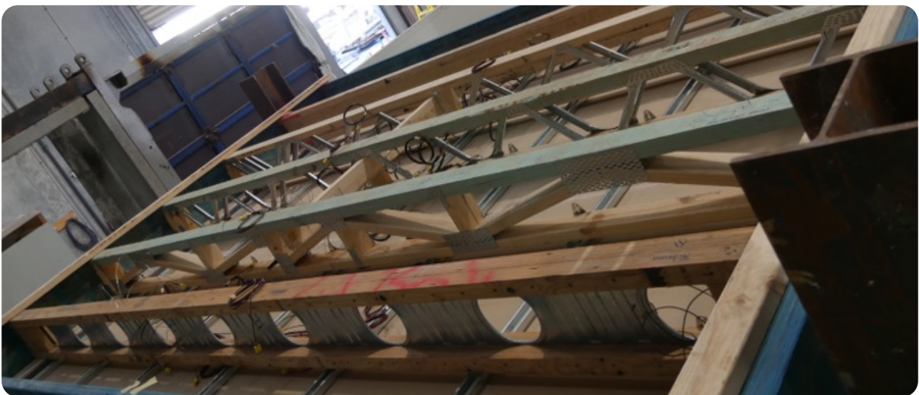
Figure 106: FRL 120/120/120 Timber floor test with lightweight engineered beam systems during construction.
