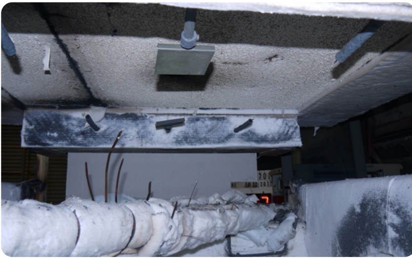
Figure 144: Post-fire test monitoring arrangement showing insulated tube mounting a heat flux meter monitoring the underside of the specimen and furnace thermocouples.
