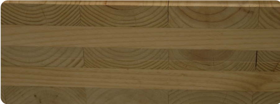
Figure 127: Edge of 225 mm thick CLT panel showing edge joints without adhesive between sides of timber sections forming the CLT panel.
