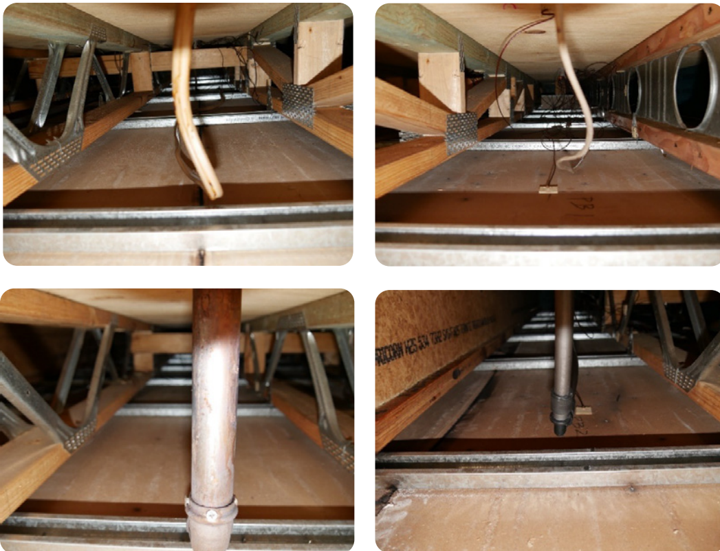
Figure 113: View within cavity showing service penetrations between beams.
