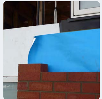
Extruded polystyrene over-cladding a timber-framed wall before external cladding is fixed.
