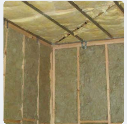
Glass-wool bulk insulation batts.
