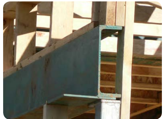
Figure 46: Thermal bridging.
