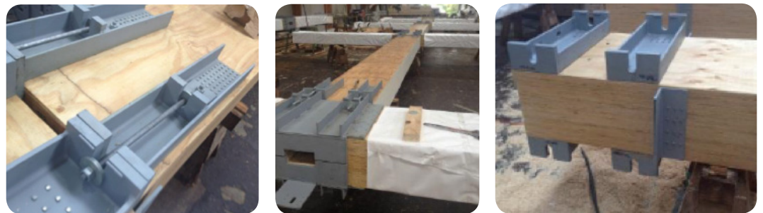
Figure 1.5: Riveted connections of the Trimble building in Christchurch, New Zealand.
