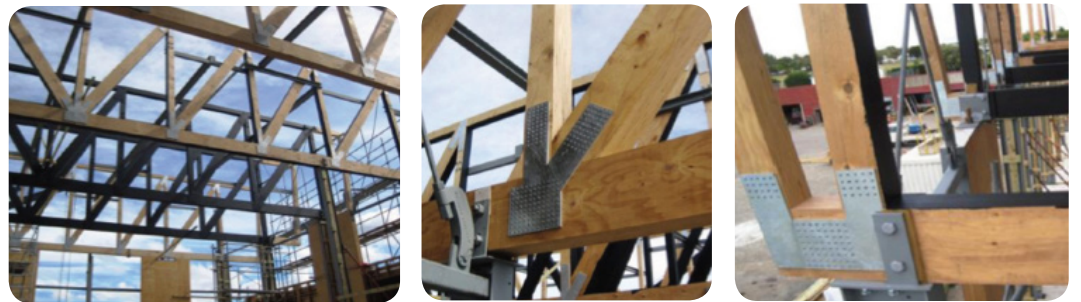
Figure 1.4: Riveted connections on the Carterton Event Centre, New Zealand.
