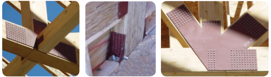
Figure 1.3: Sample applications of timber rivet connections.
