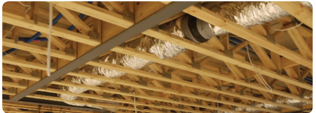
Figure 0.3: Hybrid floor system with parallel-chord trusses supported from a steel I-beam.
