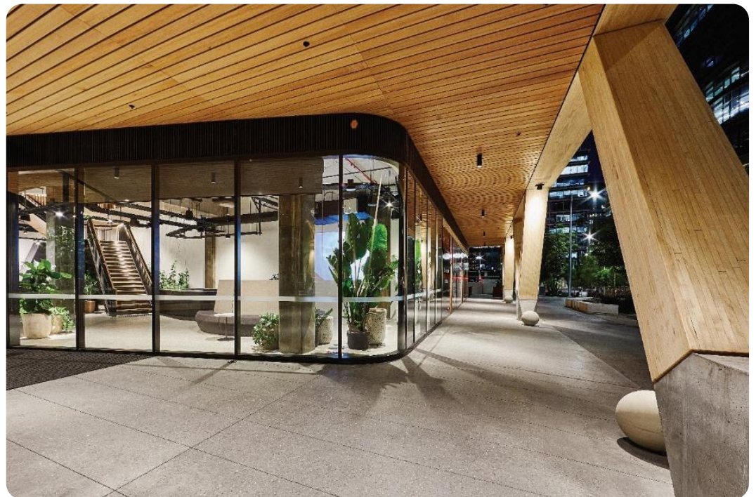
Figure 5.4: Glulam colonnade with concrete plinth bases. (Image: Lendlease)
