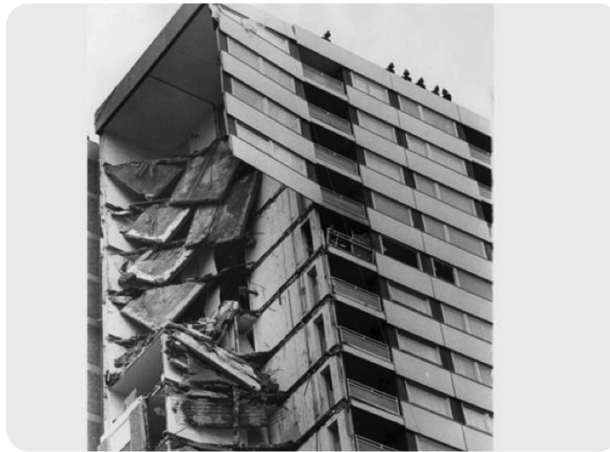
Figure 1.2: Ronan Point, UK – progressive collapse of one side of building due to gas explosion.
