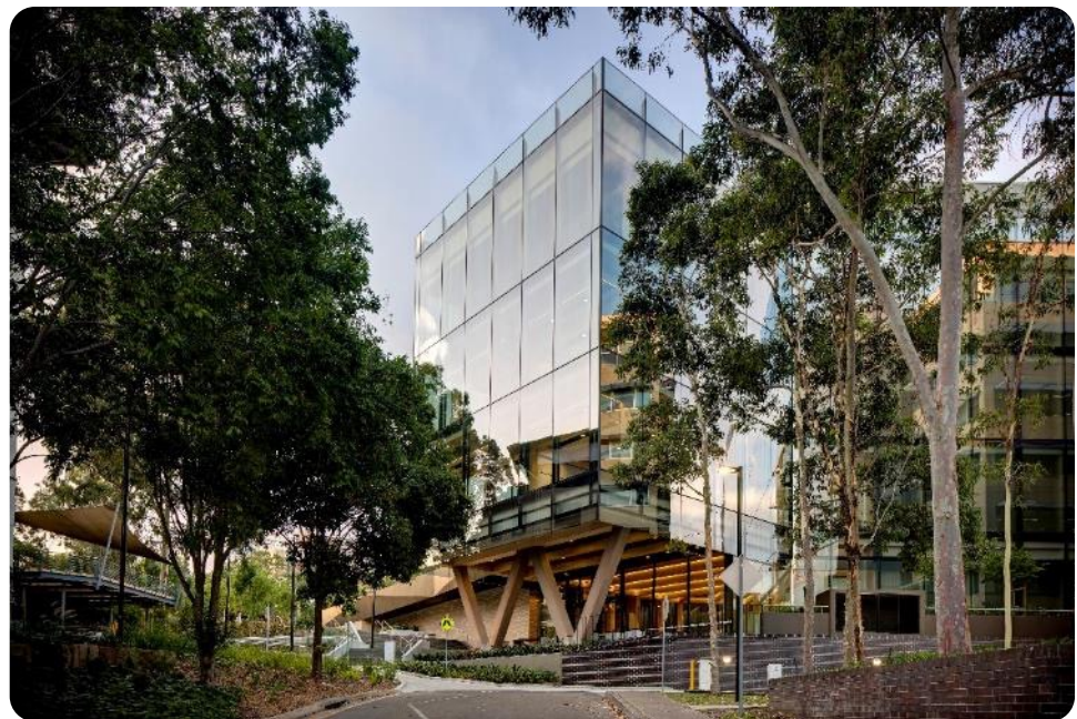
Figure 5.1: Macquarie University Ainsworth Building (Credit: ARCHITECTUS (Architects), Image: Brett Boardman Photography)
