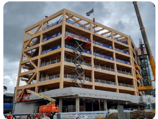
Figure 5.8: External Construction. (Image: TTW)
