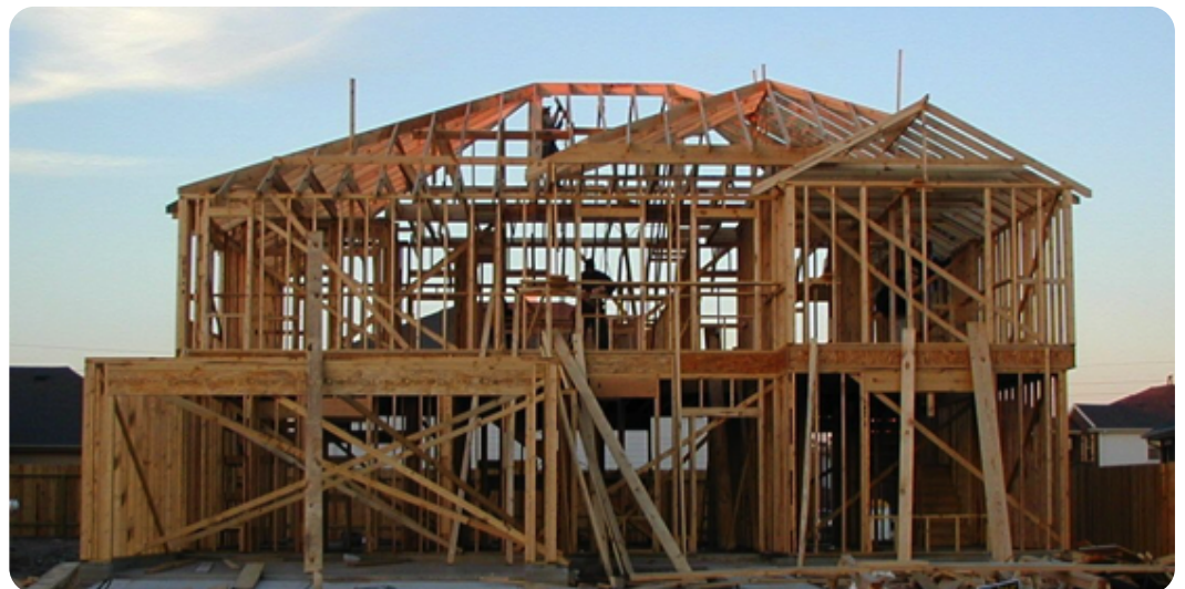
Figure 4.2: Typical timber-framed domestic construction.
