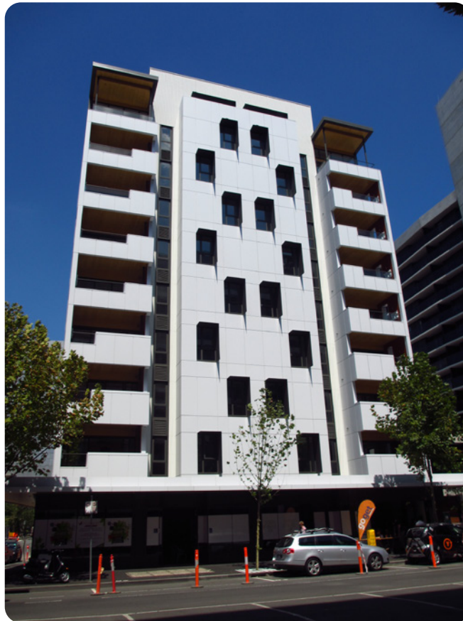
Figure 4.1: Forte, Melbourne, nine storeys of CLT on concrete podium.
