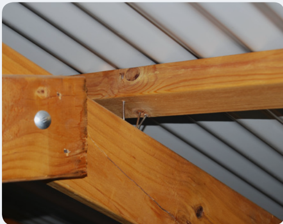
(a) Batten-to-rafter connection
