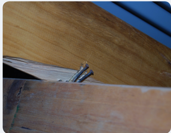
(b) Rafter-to-underpurlin connection
