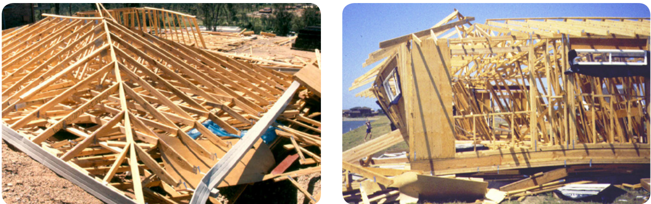
Figure 6.6: Failures of houses under construction due to inadequate temporary bracing.
