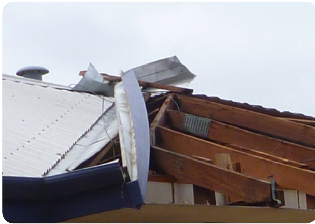
(a) Batten-to-rafter or truss connection
