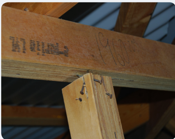
(c) Underpurlin-to-strut connection
