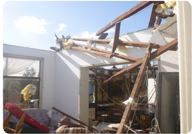
(b) Roof structure to wall connection
