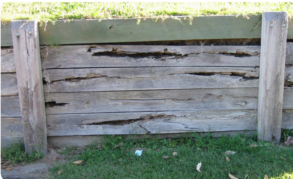
Figure 2.3: Low quality hardwood sleepers
