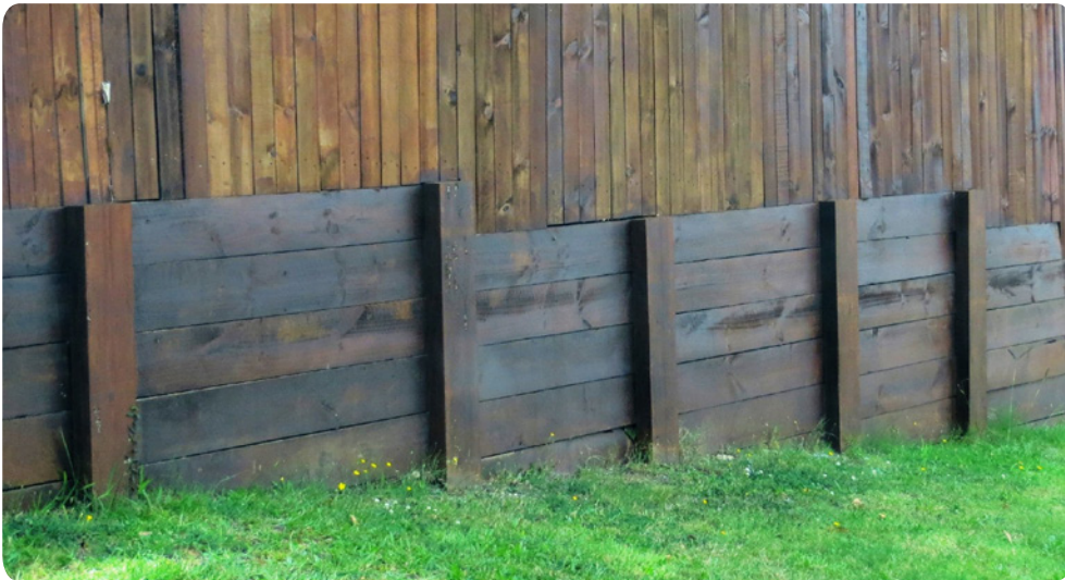
Figure 4.1: Treated pine retaining wall (and fence) being regularly maintained with application of timber preservative oil.
