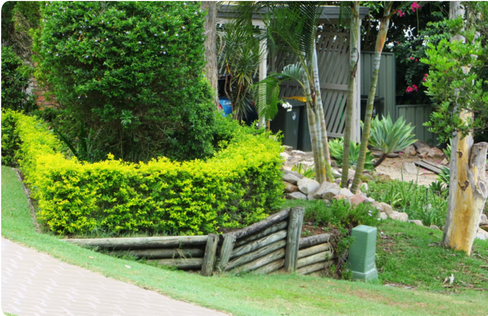
Figure 1.2: It is critical that the footing embedment of posts is adequate to prevent rotation of the posts. The treated pine rounds in this wall are still sound. The wall is failing due to inadequate embedment of posts.
