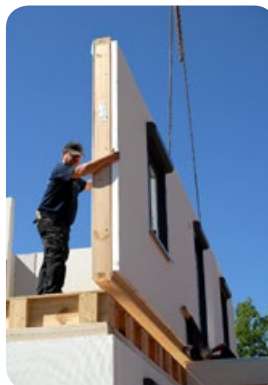
Figure 6: Prefabrication-intensive construction – panel construction.
