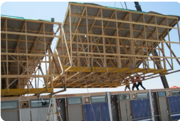
Figure 7: Site-based component assembly – roof modules
