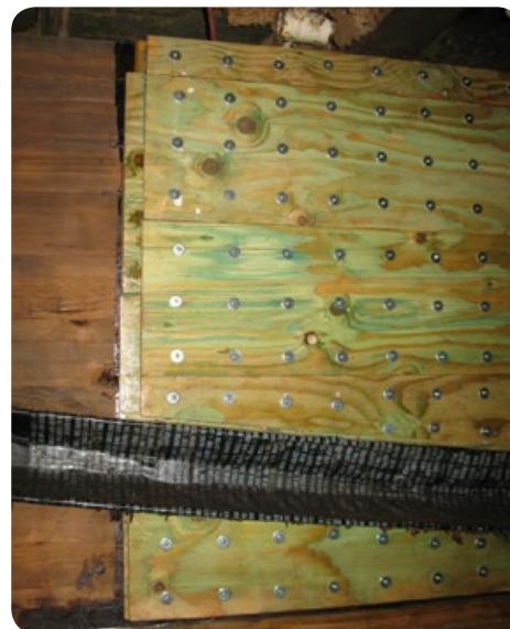
Figure 53: Example illustration of shear panels utilised around services to provide for adequate net shear resistance in the glulam element
