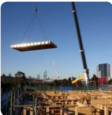
Figure 6: Prefabrication-intensive construction – panel construction.
