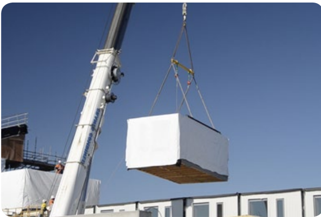
Figure 9: Prefabricated modules in installation and assembly
