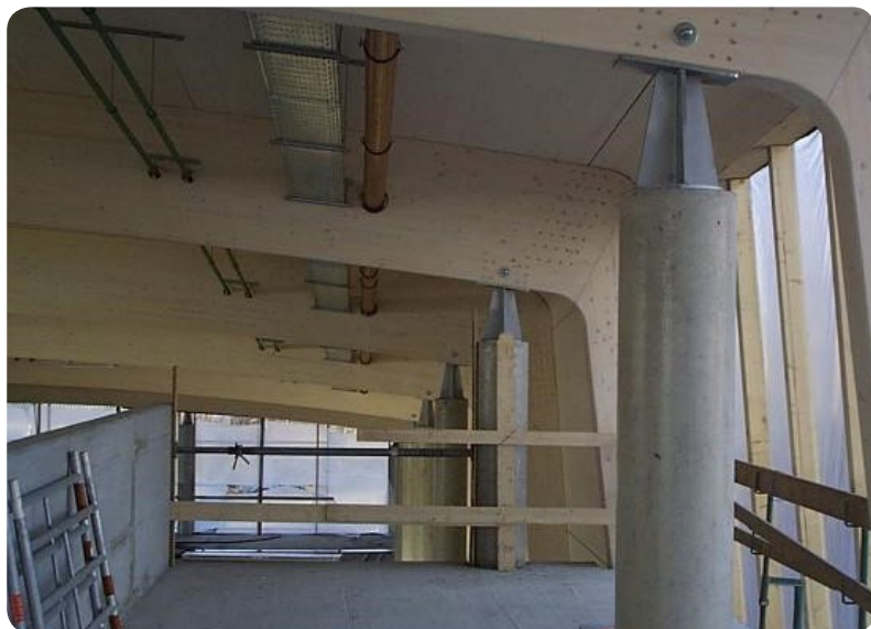
Figure 52: Example of utilities running through high strength fibre reinforced glulam beams instead of underneath such as required in unreinforced glulam
