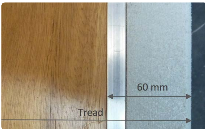
Figure 3.38. Grit-coated metal strap, 60 mm wide, at nosing of wood tread.
