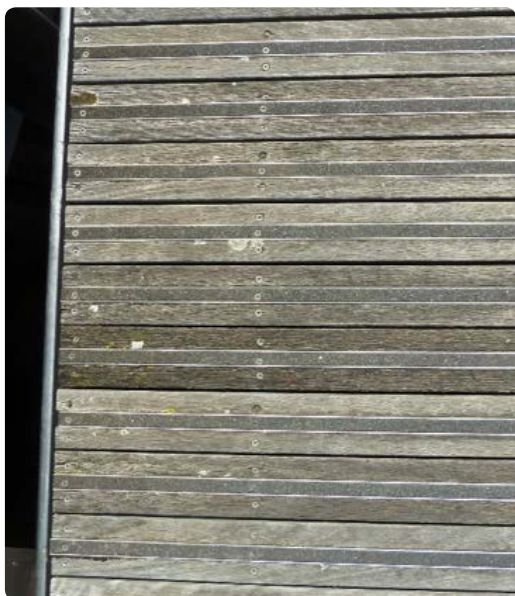
Figure 3.29: Boards with inlaid grit straps.
