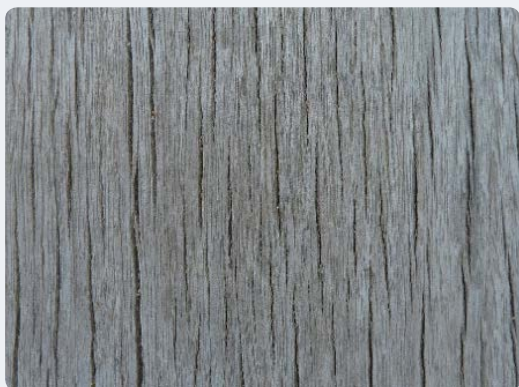
Figure 3.5: Naturally textured surface from weathering.
