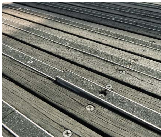
Figure 3.42: Dislodgement of inset straps.
