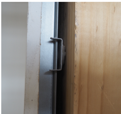
Figure 5.8 (a): Resilient mounted channel. Figure 5.8(b): Resilient channel.
