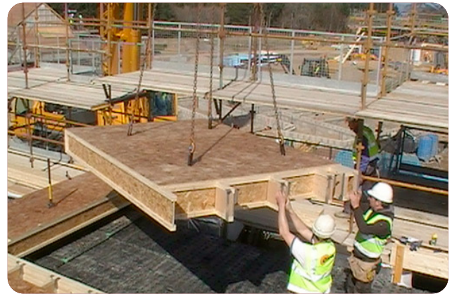
OSB or plywood
