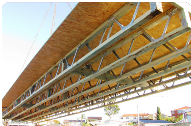
Figure 4.3: Installation of cassette floor systems.
