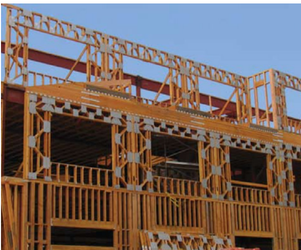
Figure 7.4: Moment-carrying frames (photograph is from USA).
