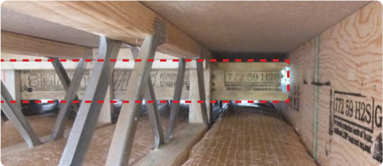
Figure 4.9: View inside a floor cassette. Note floor trusses, strong-back, edge rim-beam and also insulation. (Image TPC Solutions)
