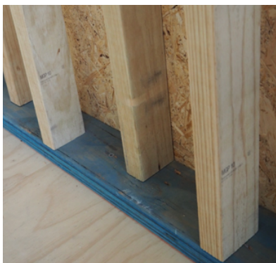
Figure 5.7: Staggered stud wall frame.
