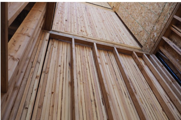
Figure 7.13: Nail laminated timber core. (Photograph: Jane Arnold, Strutterre)
