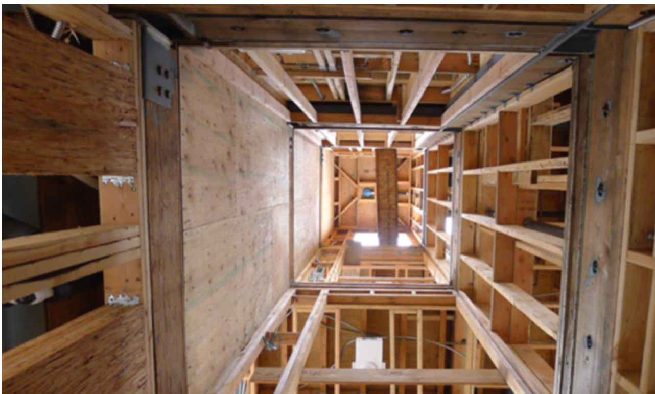
Figure 7.11: Timber-framed core. (Photograph: WoodWorks USA)
