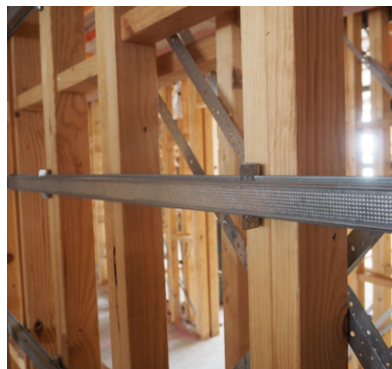
Figure 5.8 (a): Resilient mounted channel. Figure 5.8(b): Resilient channel.
