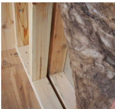
Figure 5.6: Double leaf stud wall frame.
