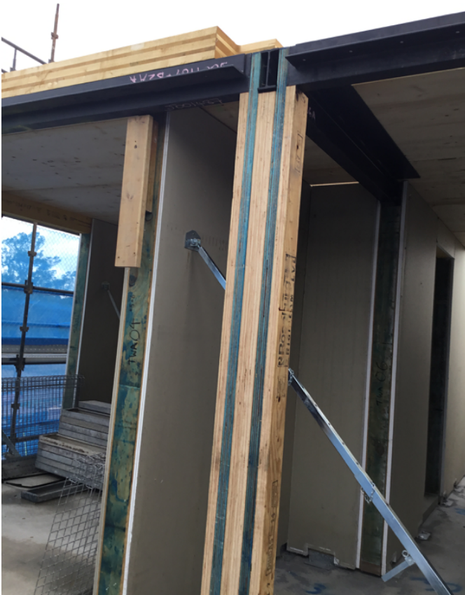
Figure 6.7: Timber studs supporting steel beam.
