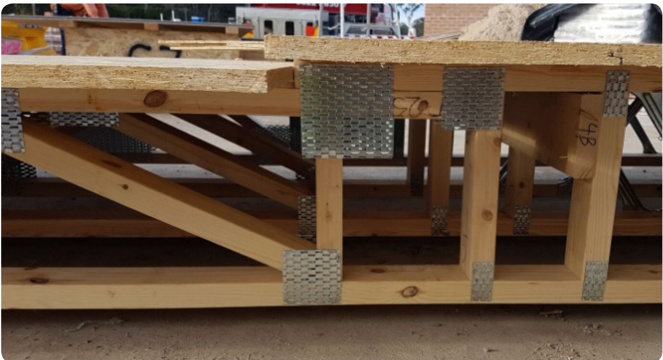
Figure 4.10: Set down formed in floor truss. (Image: TDA)
