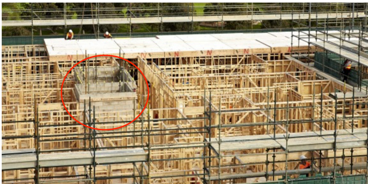
Figure 7.10: An example of a concrete core in mid-rise timber-framed apartments.
