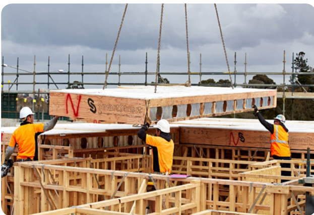
Figure 4.1: The Green (Melbourne, 2014) is a 5-storey development designed by SJB Architects (planning) and Point Architects (documentation), scaling up the traditional stud frame design and adapting it to a new set of requirements. This 57-apartment project was approved with a Performance Solution and set an example for the Deemed-To-Satisfy rules that were approved in May 2016 in the National Construction Code. Developed and built by Australand, the project reported an overall 25% cost saving with respect to the alternative concrete-based program. The advantages of timber construction in this project, according to Irwin Consult (engineers) were: 1) lighter overall building loads on columns, foundations and ground floor transfer beams; 2) reduced building mass and stiffness resulting in lower lateral design earthquake loads in comparison to concrete buildings; 3) prefabrication of walls and floor elements to achieve a construction program equal to that of equivalent concrete buildings; and 4) use of a labour force experienced with this type of construction using materials that are commonly available and economical. Images: https://citta.com.au and WoodSolutions.
