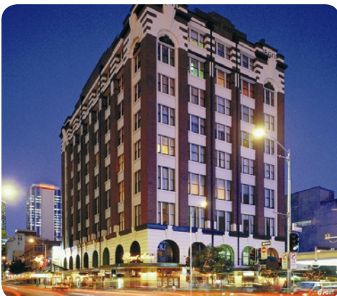
Figure 8.1: Perry House in Brisbane, a semi-tropical climate, was built in 1913 with a timber structure and masonry cladding. It was then the tallest building in Brisbane. An extra storey was added in 1923. Perry House is still believed to be the tallest timber structure in the Southern Hemisphere that's built on wooden foundations. Its timber structures were kept in the 1996 renovation and are still efficient and beautiful in its new life as the Royal Albert Hotel. Its contemporary equivalent (Figure 8.2) adopts a CNC-machined GLT and CLT structure and is clad with a glazed curtain wall, but shares with Perry House the same care in design and constructions, for a wonderful and future-proof result that makes it a valuable asset. Images: https://www.royalalbert.com.au/
