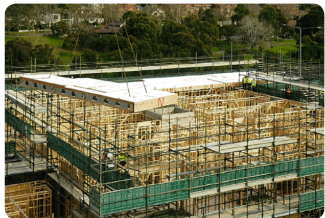
Figure 4.1: The Green (Melbourne, 2014) is a 5-storey development designed by SJB Architects (planning) and Point Architects (documentation), scaling up the traditional stud frame design and adapting it to a new set of requirements. This 57-apartment project was approved with a Performance Solution and set an example for the Deemed-To-Satisfy rules that were approved in May 2016 in the National Construction Code. Developed and built by Australand, the project reported an overall 25% cost saving with respect to the alternative concrete-based program. The advantages of timber construction in this project, according to Irwin Consult (engineers) were: 1) lighter overall building loads on columns, foundations and ground floor transfer beams; 2) reduced building mass and stiffness resulting in lower lateral design earthquake loads in comparison to concrete buildings; 3) prefabrication of walls and floor elements to achieve a construction program equal to that of equivalent concrete buildings; and 4) use of a labour force experienced with this type of construction using materials that are commonly available and economical. Images: https://citta.com.au and WoodSolutions.
