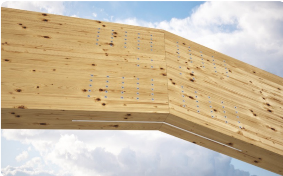
Figure 49: Dowel used in a joint in a large timber truss. (Image credit: Rothoblaas)
