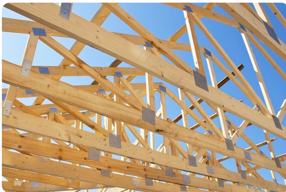
Figure 3: Timber nail plate truss. (Image credit: MiTek)
