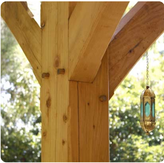
Figure 48: Modern timber dowel joint. (Image credit: Australian Timber Frame)
