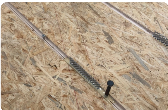
Figure 88: Glued-in shear connectors in a timber-concrete composite floor panel. (Image credit: TDA)
