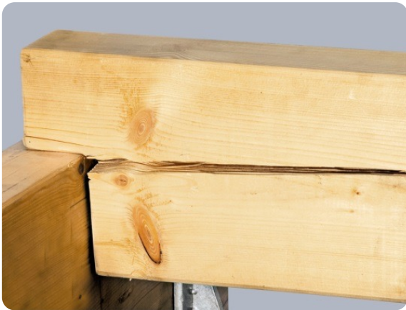
Figure 32: Modern screw reinforcing a notched beam. (Image credit: Spax)
