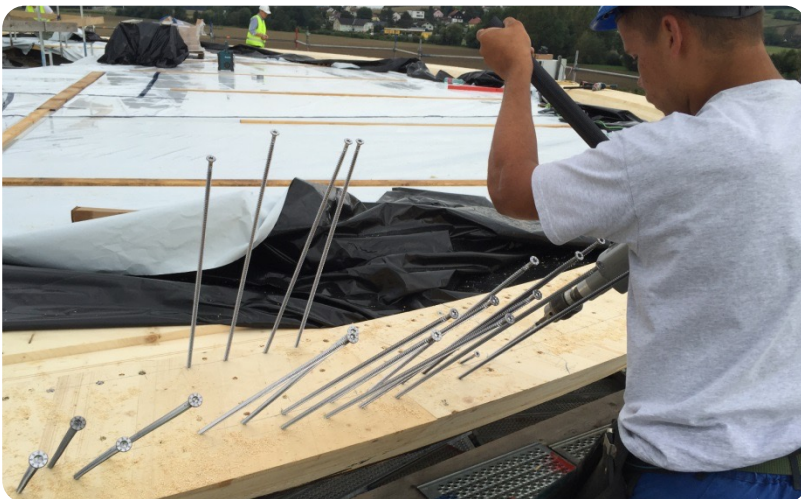
Figure 30: Long screws used in construction. (Image credit: TDA)
