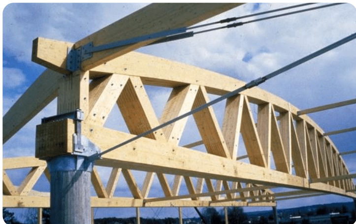
Figure 73: Main truss of the Hamar Olympic Amphitheatre, Norway. The span is 71 m. The truss nodes consist of nine slotted-in plates and dowels. (Image credit: Moelven Limtre A/S).
