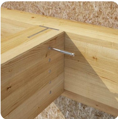
Figure 77: Self-drilling dowels T plate connector. (Image credit: Rothoblaas)
