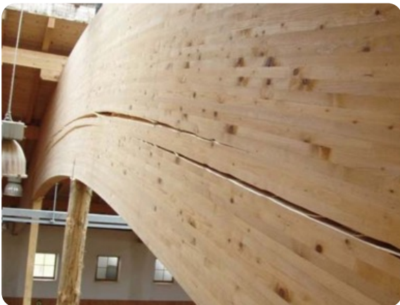
Figure 33: Reinforcement of curved glulam. (Image credit: Spax)
