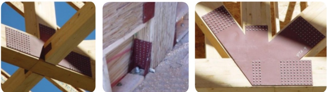
Figure 82: Application of Timber Rivets. (Image credit: Specialized Timber Fasteners Ltd, Canada)
