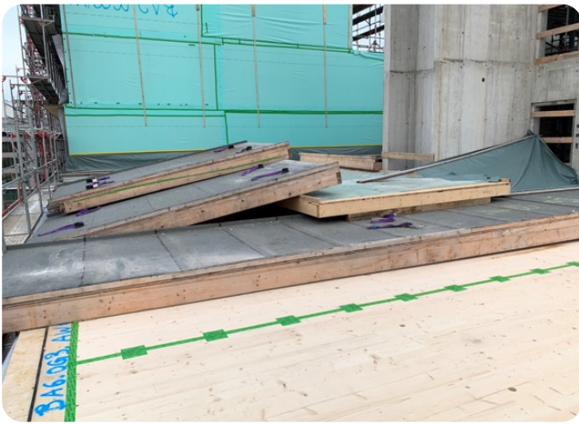
Figure 28: Temporary roof panels awaiting installation. (Image: TDA)
