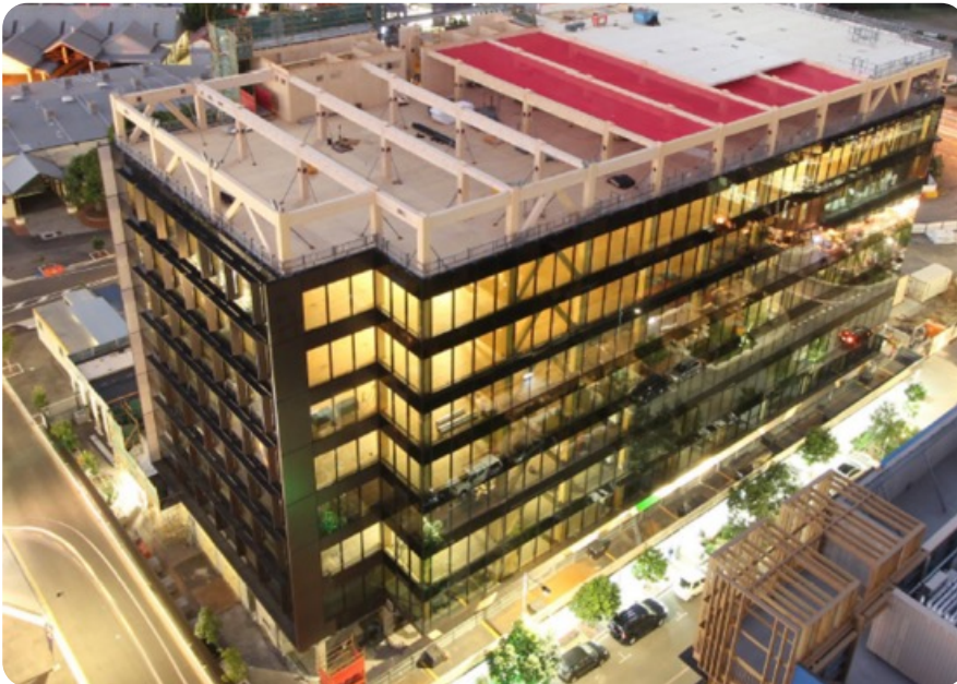
Figure 18: Façade enclosing the building aiding in weather protection. (Image: Tom Roe)
