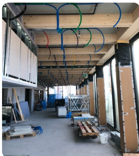
Figure 26: Protection of mass timber columns. (Image: TDA)
