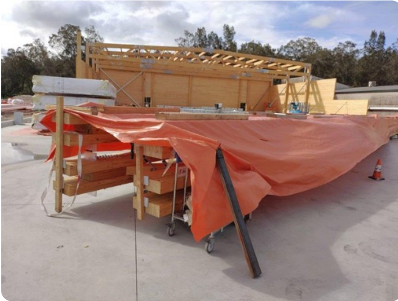
Figure 20: Impermeable covering with a respectable spacing of timber elements and airflow. (Image: CWC)
