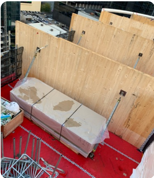
Figure 27: Vapour permeable membrane fixed to CLT floor panels. (Image: TDA)
