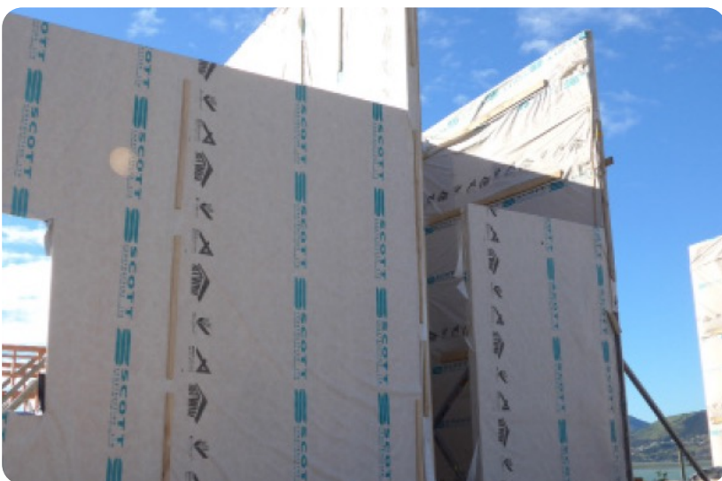
Figure 21: Wrapping left in place to protect the timber element. (Image: XLam Australia)
