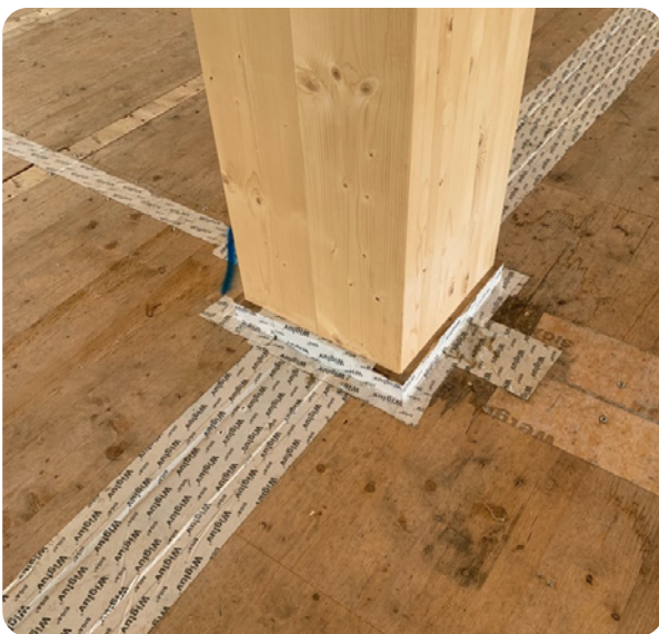
Figure 22: Tapes used to cover joints in CLT floors.
