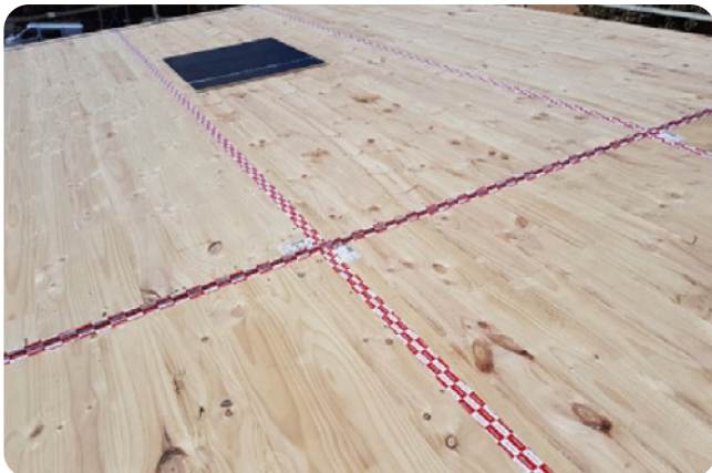
Figure 25: Tape used to seal joints and end grain. (Image: XLam Australia)
