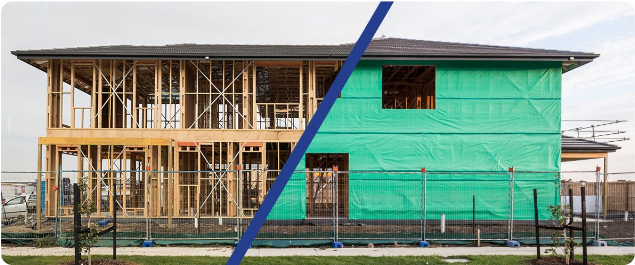
Figure 13: Reverse building practices weather-tight the building at an earlier stage. (Image: Bradford Insulation)
