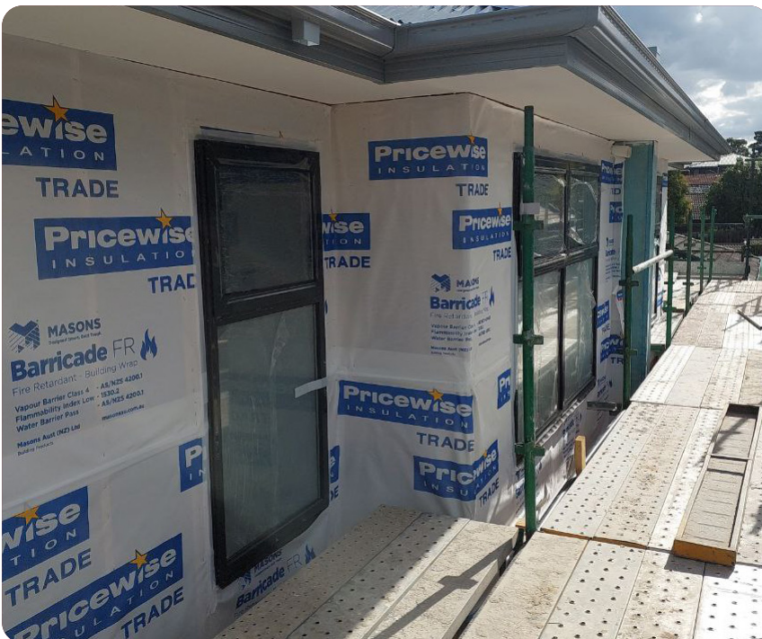
Figure 14: Sarking-wrapped house. (Image: Pricewise Insulation)
