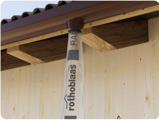
Figure 16: Temporary downpipes. (Image: Rothoblaas)
