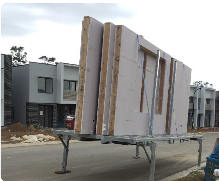
Modular wall panels delivered to site, Phoenix Building, Sydney, NSW. Image source: TPCSolutions
