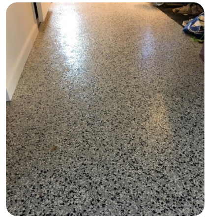
Figure 24c: Epoxy finish on a concrete floor (Image Credit: JDA)
