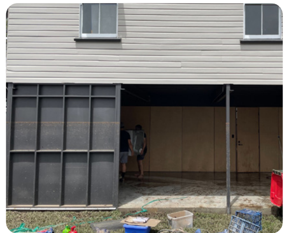
Figure A10: Wilston House immediately after the February 2022 flood. The single skin walls meant there were no cavities for the flood waters to enter and be trapped. (Image Credit: JDA)
