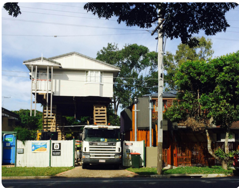
Figure 30: A house being raised on temporary styes (box cribbing or cribbing blocks). (Image Credit: JDA)
