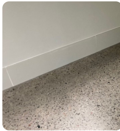
Figure 24b: Polished concrete floor well sealed (light grind) (Image Credit: JDA)
