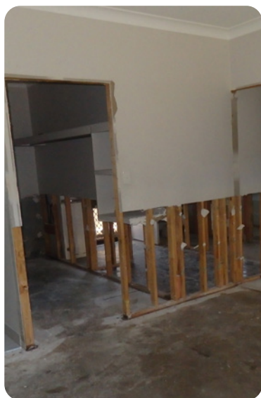
Left: Figure 16: Timber wall frames are partially stripped to the nearest set joint in the wall lining to facilitate sanitary works and drying. (Image credit: JDA)
