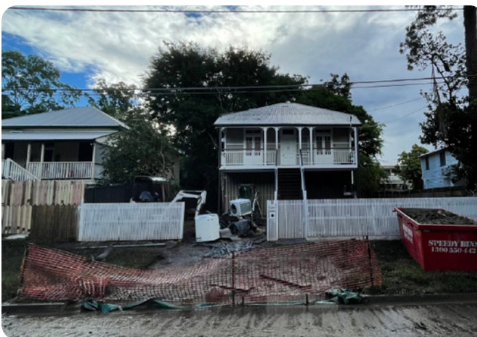
Figure A11: Permeable fencing at the front of the property meant that water could flow through without damaging the fence. (Image Credit: JDA)
