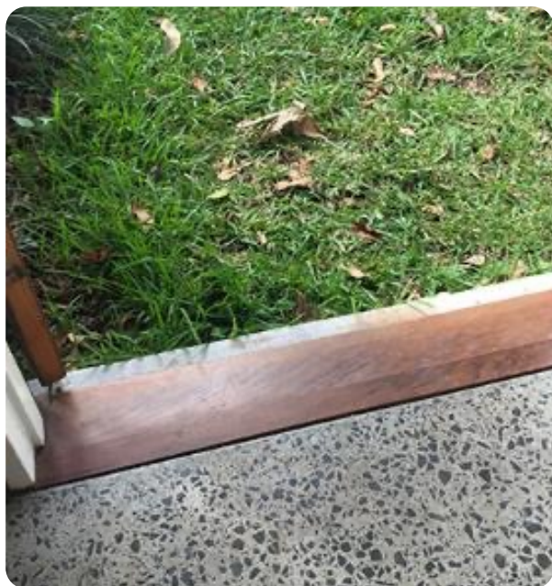
Figure 25: Flush door sills (Image Credit: JDA)
