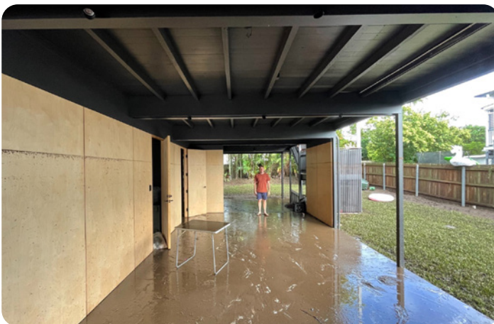
Figure A10: Wilston House immediately after the February 2022 flood. The single skin walls meant there were no cavities for the flood waters to enter and be trapped. (Image Credit: JDA)
