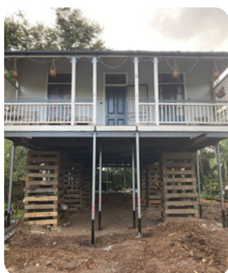
Figure A8: Wilston House during and after the raise. (Image Credit: JDA)
