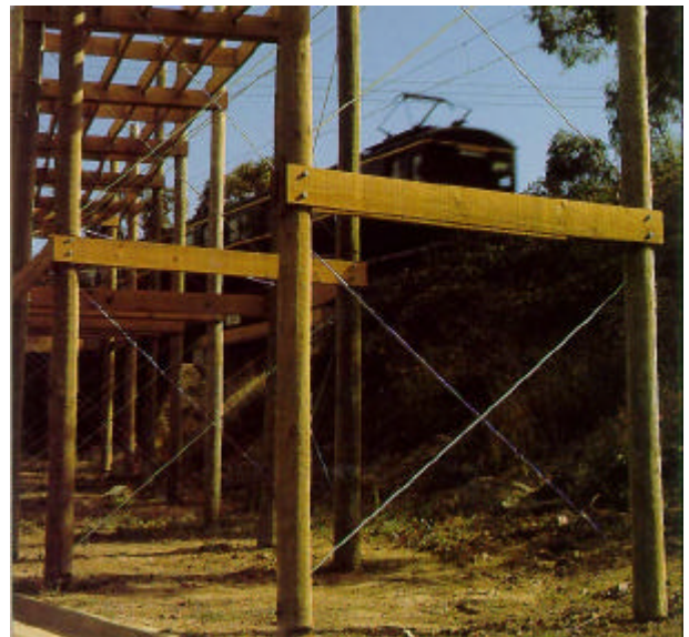
Simple bolted joint between beams and poles provide supporting structure for pedestrian bridge
