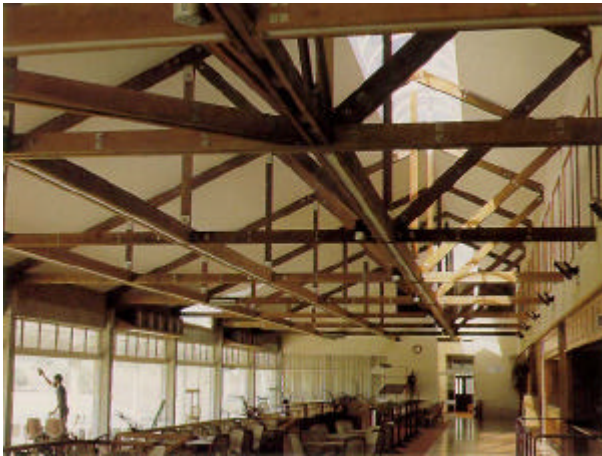
Exposed heavy timber bolted trusses provide clear span and airy atmosphere for food and beverage facility
