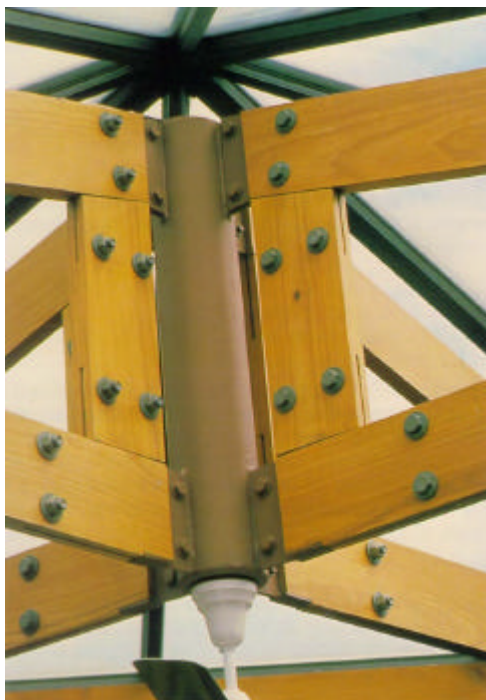
Bolted trusses fixed to central metal connector in school roof structure
