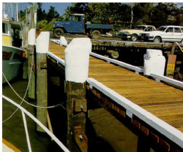
Heavy hot dipped galvanised bolts connect timber wharf structure
