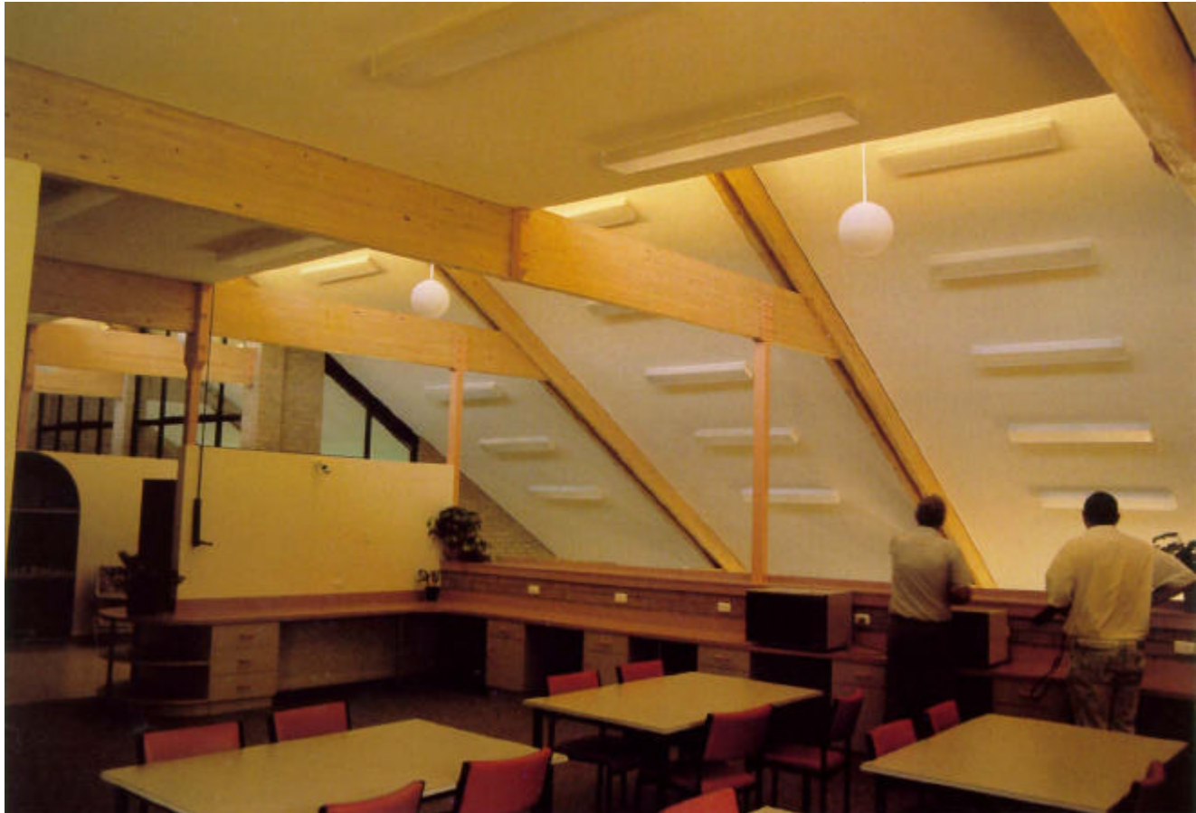
Simple bolted joints in glued laminated beam roof structure
