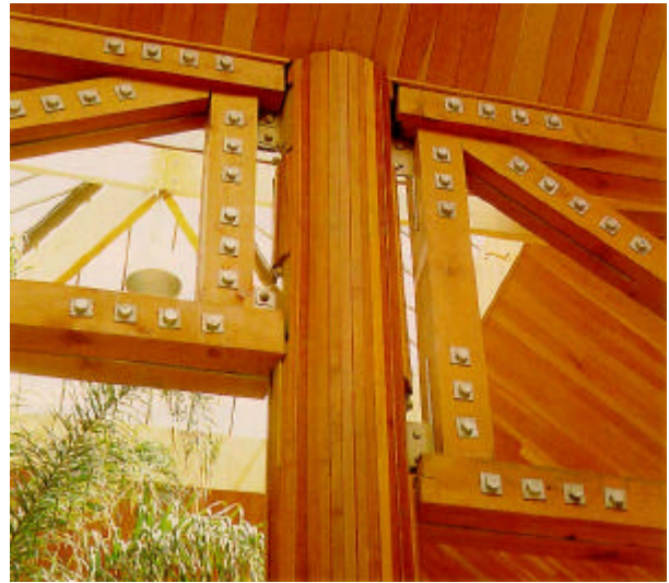
Trusses featuring bolts and large washers in shopping complex
