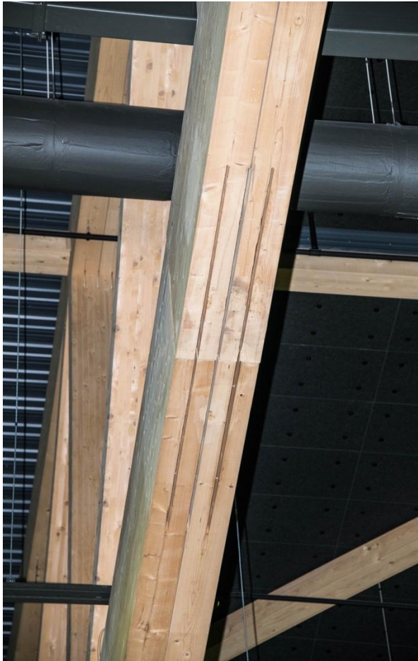
Figure C1(a) Slotted plate tension connection
