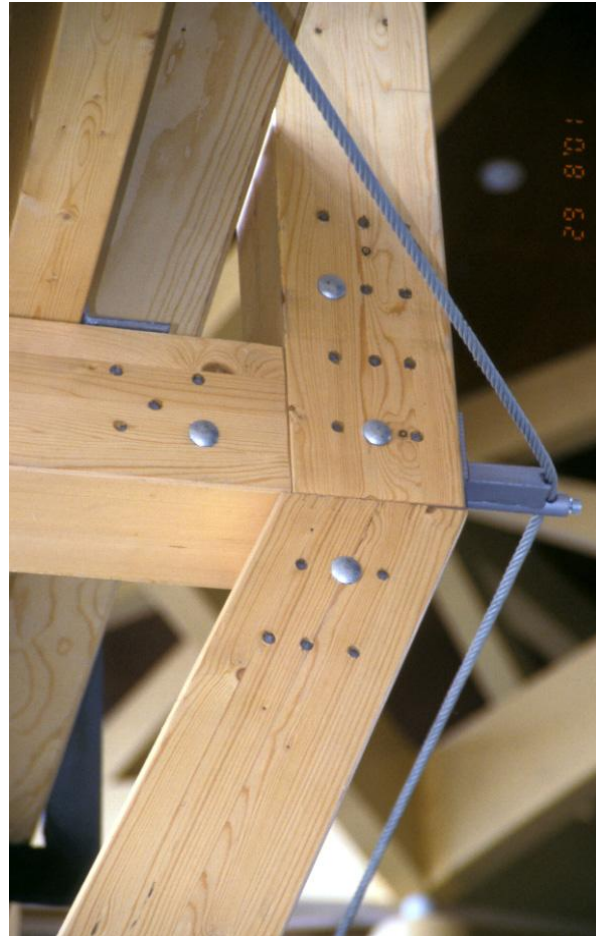
Figure C1(b) Concealed slotted plate tension connection
