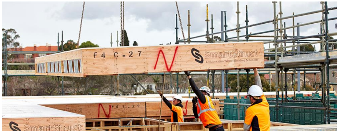
Image: Installation of the cassette floor system for the Green
