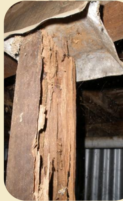
Termite damage to a timber stump
