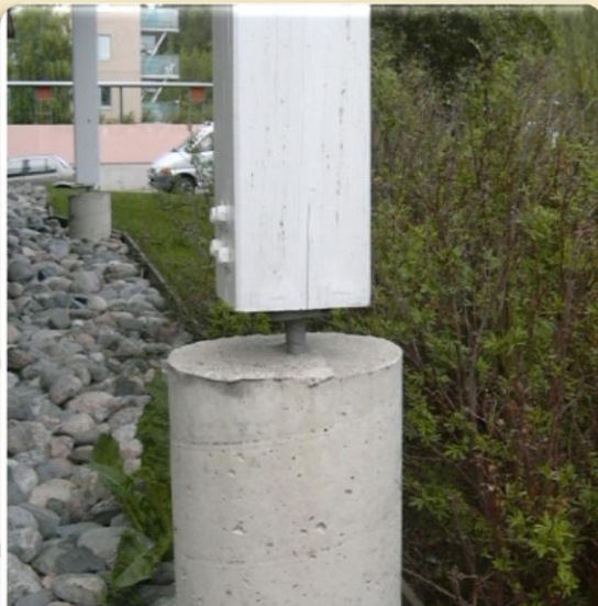
A well-ventilated, free-draining post support.
