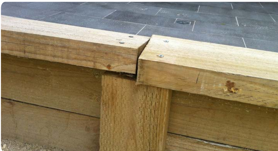
Figure 3.7: Inadequately fixed (screws of insufficient length) resulting in distortion (twisting) of sleepers used on flat.
