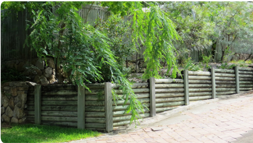
Figure 2.1: Combination of durable hardwood posts and H4 CCA treated rounds
