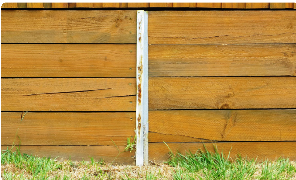
Figure 2.5: Poor quality galvanized steel 'H' section post showing corrosion approximately 8 years after installation
