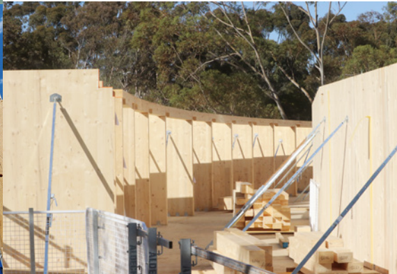
La Trobe University, JCB Architects
