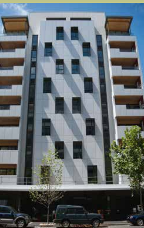
Forte – Australia's first CLT building constructed by Lend Lease
