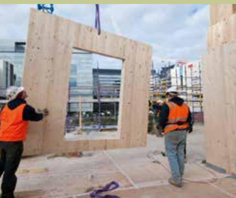
CLT wall panel installation at the Forte project in Melbourne
