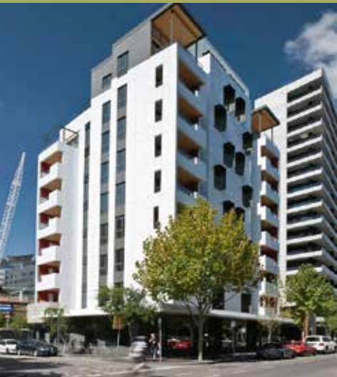
Forte – Australia’s first CLT building constructed by Lend Lease
